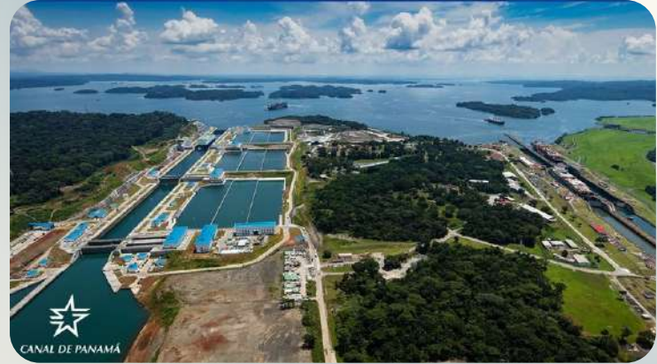
Panama Canal Expansion Program [Photo Courtesy of Canal de Panama]
